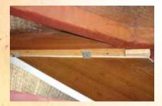
5.4 The cut should be half the wood piece, leaving the excess to place the next roll.
