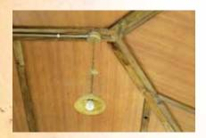
8.1 Install the lights using pipes or chutes; you can dye them using the same color of the wood to give a better appearance to the electrical installation.
