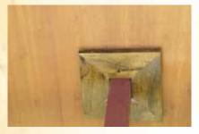
7.1 With 2" boards, make a square with cuts at 45 degrees and fasten them to the ceiling structure.
