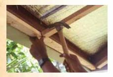
2.2 Assemble the boards with  $1 \frac{1}{2}$ " nails; use a  $1 \frac{1}{2}$ " drill tip to fasten to the cold rolled C section, if necessary.
