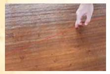
3.1 With a line drawer, draw the structure you want to add the finish to. For instance, the edge of a corner should always have an excess of 5 cm. to the measurement you want to cover, to make the piece adjustment easier.
