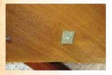
4.2 Use the head screws for the ceilings or build small 1" x 1 " tin squares to fasten the insulation to the wood of the frame skeleton across the structure. Remember that you will have flexibility with the placement of the PRODEX Rustic<sup>®</sup> so that you can get the proper position thanks to the over measurement of the initial cutting.
