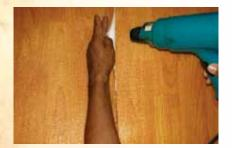
6.1 PRODEX Rustic<sup>®</sup> has a 3 mm thermo-welded platform to join the overlaps of two rolls, if necessary. This process is carried out by applying heat to the edges of the foam that are exposed and pressing a little with the palm of your hand; with this type of joint, the completely impermeable mechanical seal is guaranteed between both rolls.
