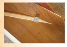
5.3 Remove the excess PRODEX Rustic<sup>®</sup>, this is the over measurement left at the beginning of the installation.
