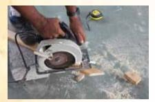
2.1 With 1  $\frac{1}{2}$ " x  $\frac{1}{2}$ " wood board, make a frame skeleton with a configuration of 1.20 meters of distance between boards; these will be the points where the rolls of Prodex Rustic<sup>®</sup> will be installed.
