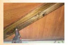
6.2 Screw the 2" wood piece on the frame skeleton by covering the fastening pieces and the joints of the rolls of PRODEX Rustic<sup>®</sup>, using a 2" fine tip screw.
