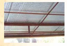
1.1 Make sure the distance between the drivers is not smaller than 2 meters between each support; otherwise, install extra pipes to obtain a proper distance and avoid future undulations on the material.
