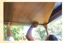
4.1 Once the PRODEX Rustic<sup>®</sup> is placed, fasten it to the frame skeleton by placing a fourth round board on top so that the board acts as a support and pressing at the same time; therefore, you can handle the PRODEX Rustic<sup>®</sup> and get the required position.
