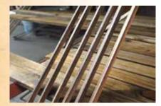
1.3 For the edges, use  $\frac{1}{2}$  rods of four round, consider 35 linear meters per each 100 square meters of ceiling.
