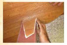
5.1 In case there are two columns in the place where the structure will be placed, cut and try to obtain the same shape as that of the PRODEX Rustic<sup>®</sup>.
