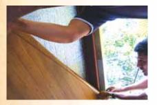
5.2 With the line drawer, draw a mark in the middle of the wood beam to which the Prodex Rustic<sup>®</sup> was fastened.
